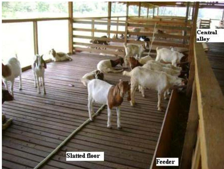
Figure 16. A slatted floor, semi-open barn with feeding trough and a central alley
